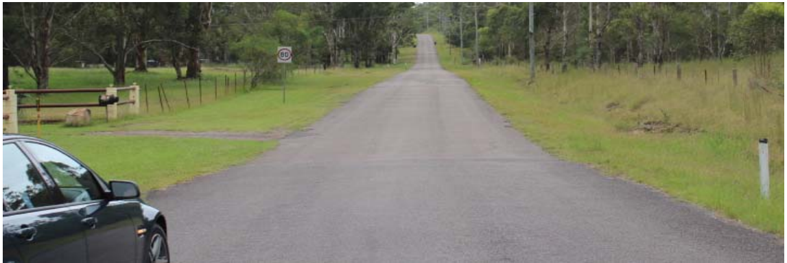
Figure 3-12 – Six Mile Road facing east near Newline Road
